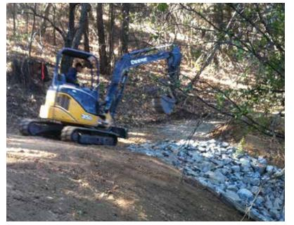
Mann Excavating improves a stream crossing on the Dunn-Wildlake Preserve road system as part of a water-quality-focused erosion control project within the Bell Canyon Creek watershed.
